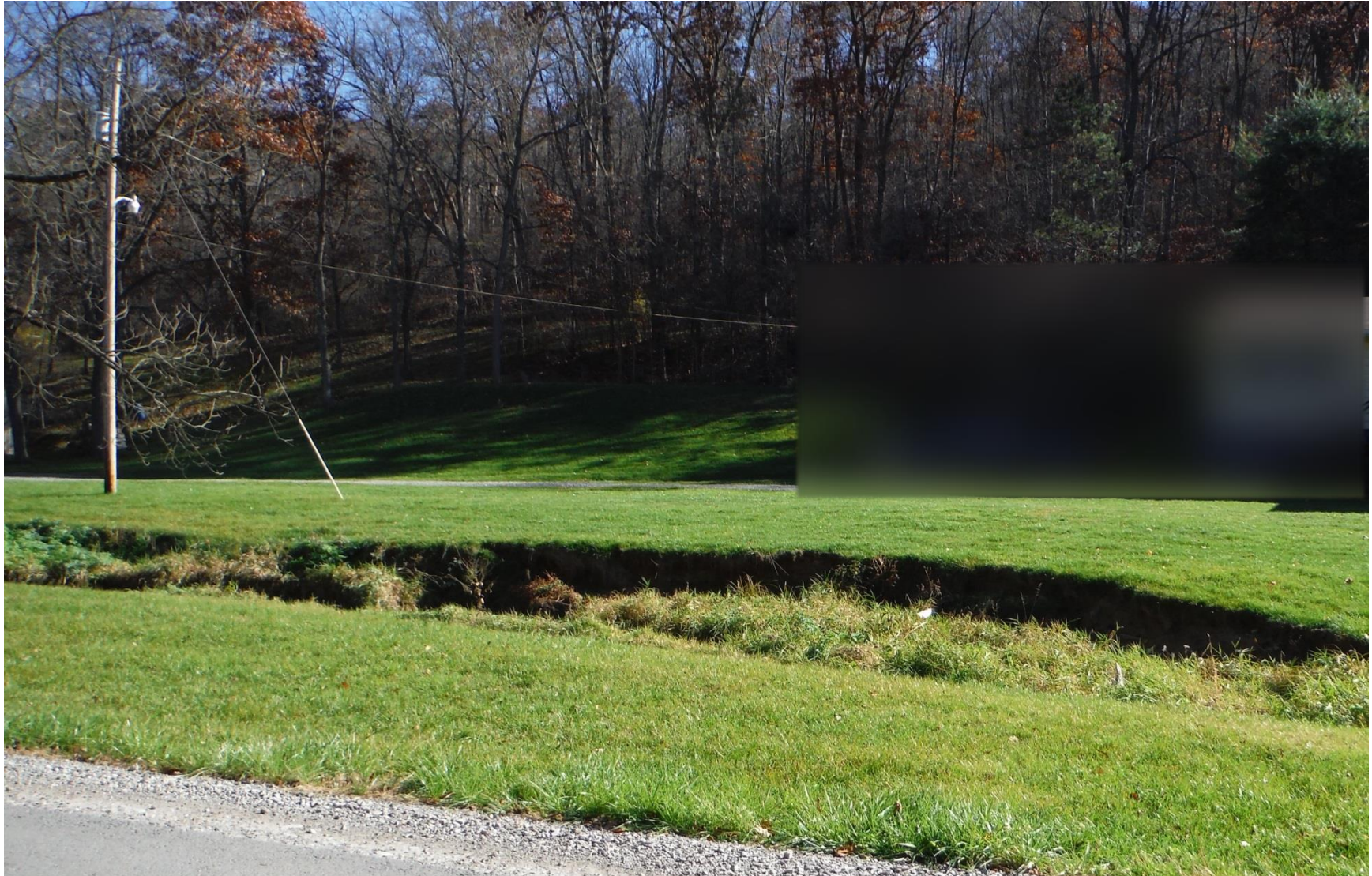
Again, the banks at this site are highly eroded due to lack of riparian vegetation. Water quality at this site would benefit from bank shaping and development of riparian buffers. Parts of this image have been obscured to preserve landowner's privacy.
