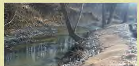
Whiteley Creek Stream Restoration Project being completed by Iron Cumberland, LLC
