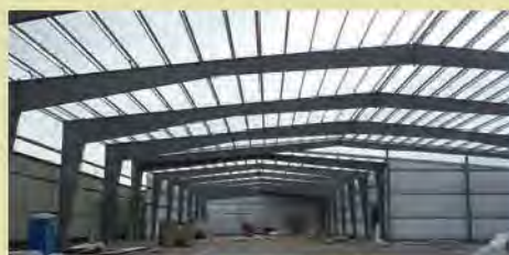
Universal Belting Resource Building Expansion in Paisley Park, Carmichaels
