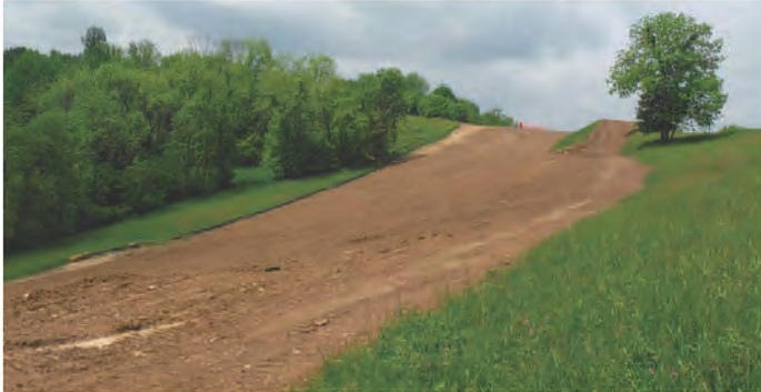
A good example of stabilizing earth disturbance to help stop accelerated erosion.
