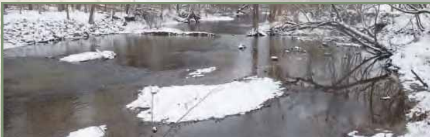
This post-construction photo shows the creek flowing unobstructed through its original channel. Recycled concrete from the removed bridge has been placed along the southern bank to strengthen the slope and prevent future erosion. The site is now safer, more stable, and more ecologically resilient.
