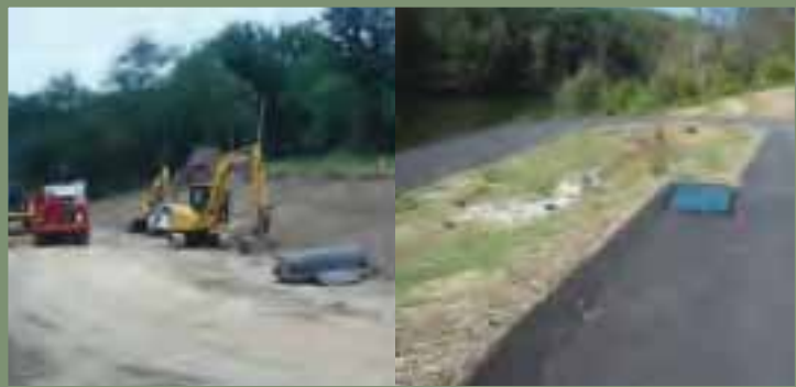
Wisecarver Park during different stages of construction
