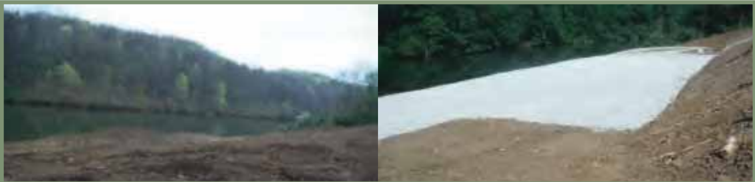
Wisecarver Park during different stages of construction
